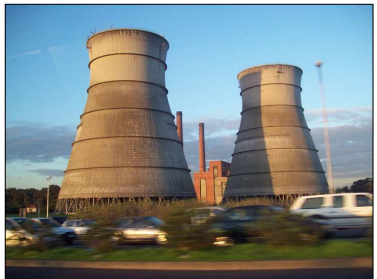
Cooling towers in South Africa [ACTSA]
